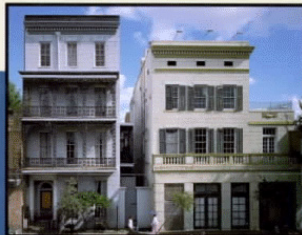
The same two buildings, 1993
