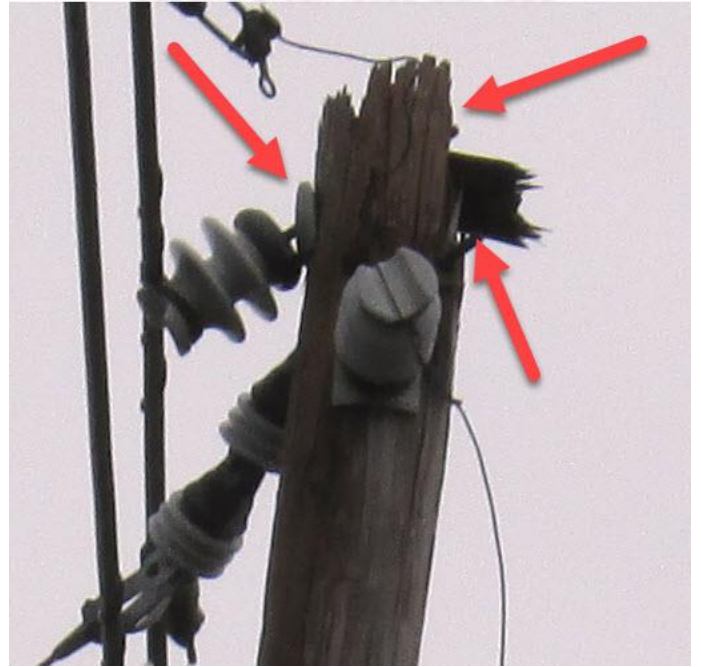
Creosote older than 40 yrs will hollow out and break loose with load
