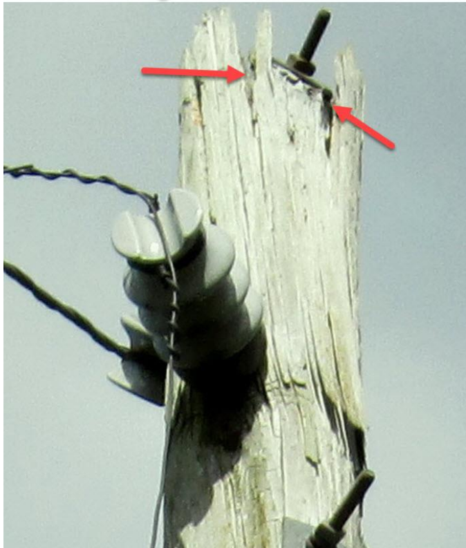
Early 80s CCA. top can not hold weight of conductor
