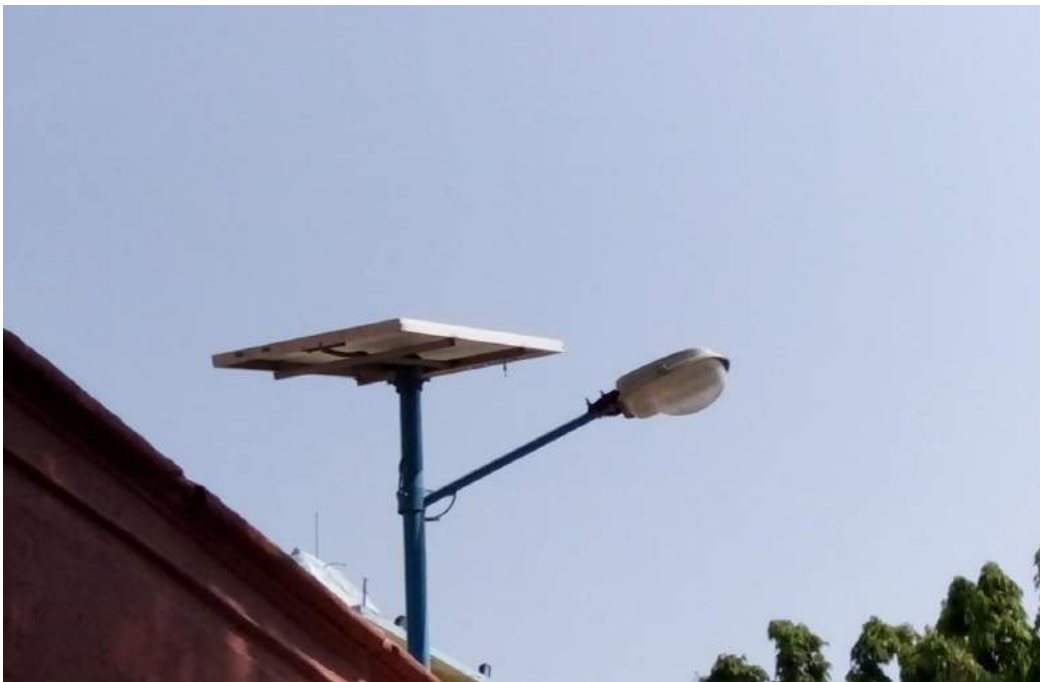
Installation of Solar Street lights
