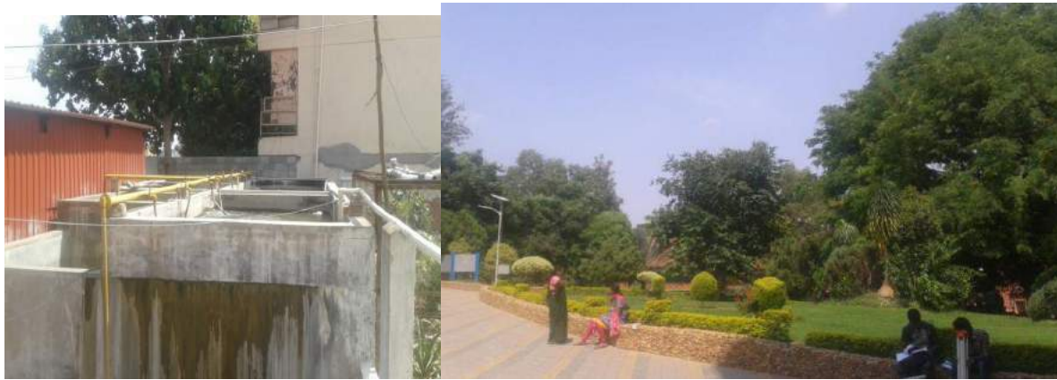
Picturesque View of Greenery managed by recycled water
